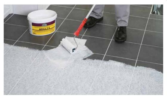
The consistency of ARDEX P 4 Primer virtually eliminates drips and splashes, making it ideal for use on walls, ceilings and floors, on a wide range of absorbent and non-absorbent substrates.
