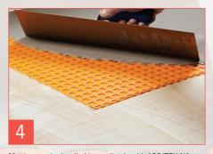
Matting can be levelled immediately with ARDITEX NA, to quickly and easily create a flat, level surface.
